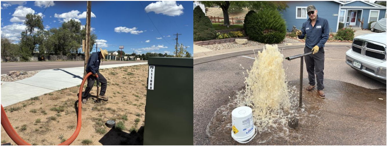
(Left: Jairo Pineda vacuuming out a valve box. Right: Jairo opening a blow-off to start a dead-end flush)
