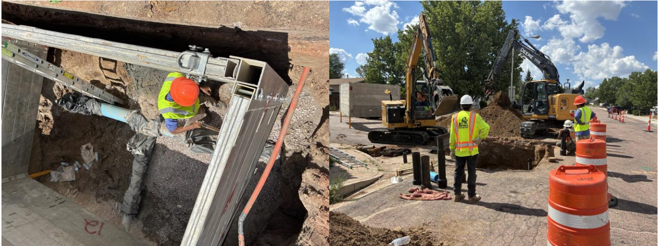
(RJ Gleeson's crew setting up the valve cluster at Omaha and Winnebago)
