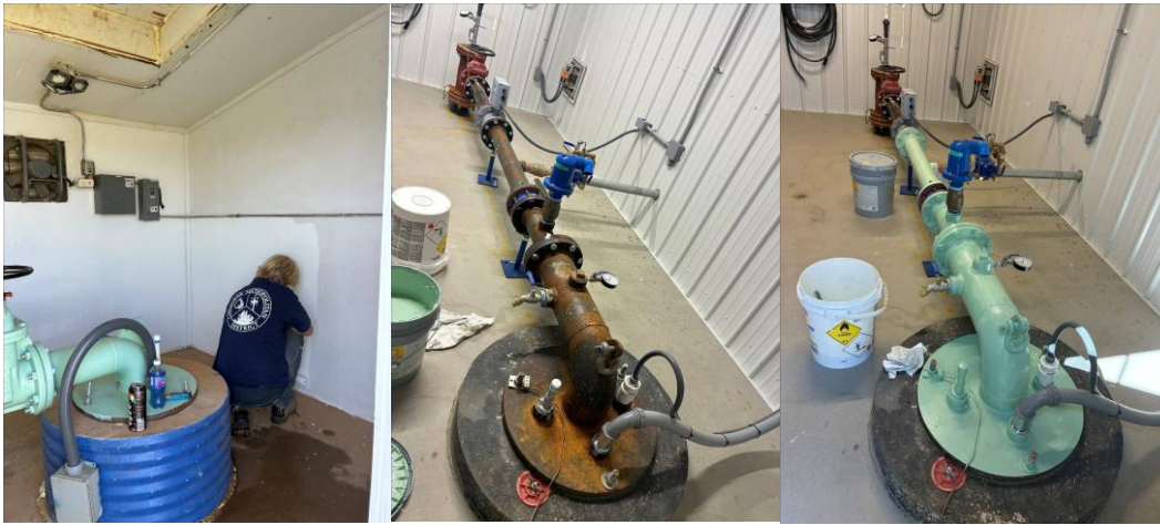
(Left: Max Heet repaints and seals one of our South wells. Center and Right: Well 22, before and after painting.)
